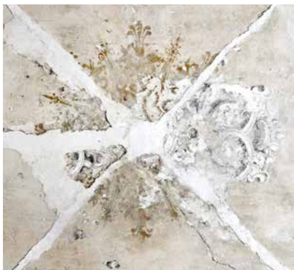
10. Central part of the ceiling in the palace at Novi trg 4 during the uncovering and documenting of several painted layers, photo by Tjaša Pristov, 2011
