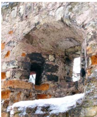
Loophole without a special gun support in the middle cavity in the city wall at the Rūdninkai Gate in Vilnius. View from the side of the city
