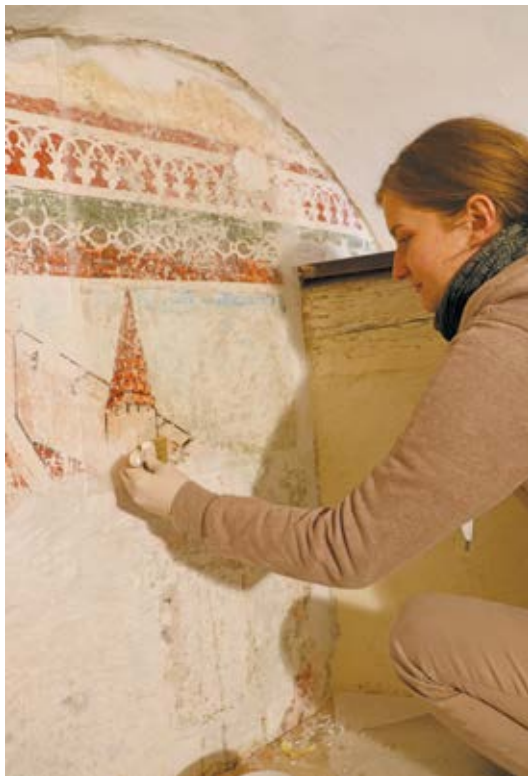
11. Application of nanolime by brush over Japanese paper, photo by Eva Marija Fras, 2020
