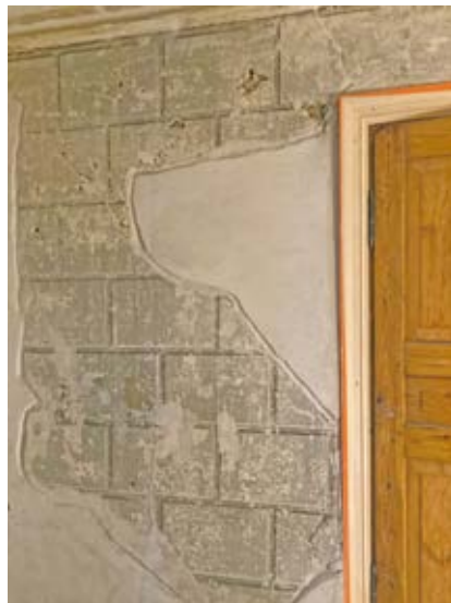
7 B. A fragment of rustic décor shortly before completion of restoration works. Photo by Rūta Astasevičiūtė, 2021
