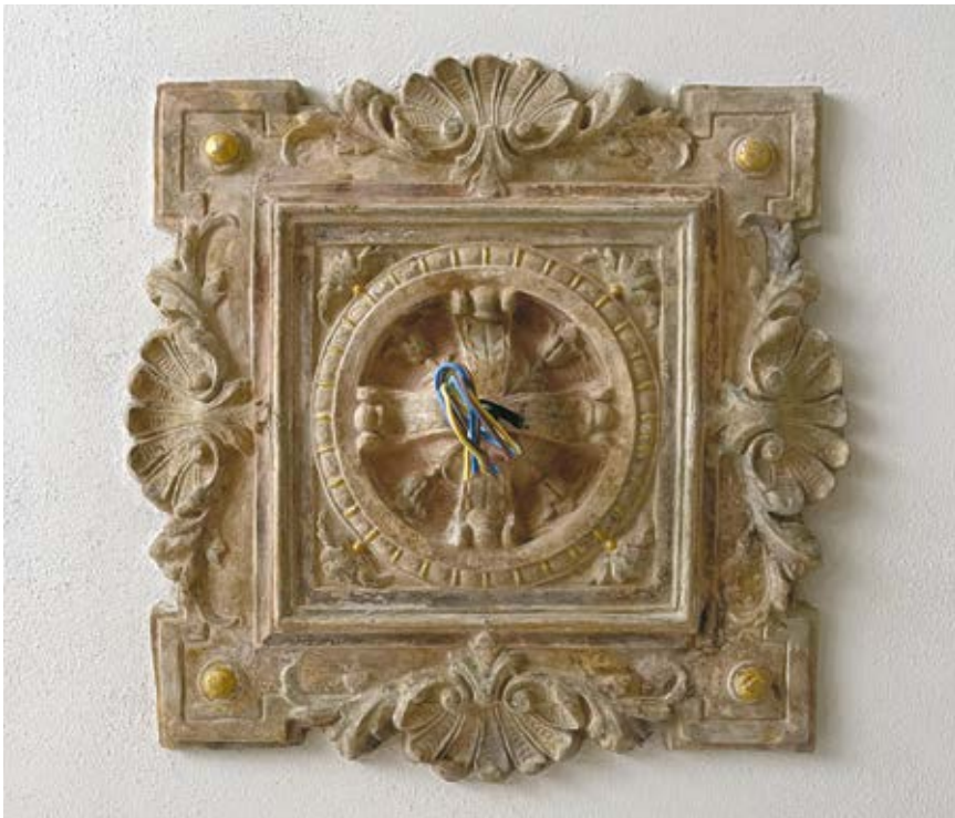
6 B. Rosette in the room on the attic after restoration. Photo by Vilius Mateika, 2022
