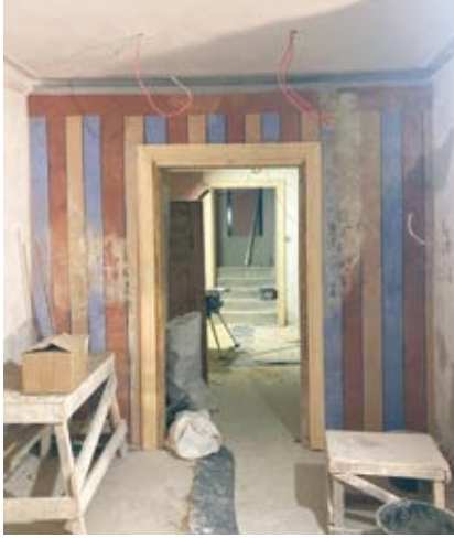
8 A. Polychrome decor of the lobby during restoration
