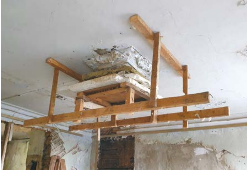
6 A. Rosette in the room on the attic during restoration works. Photo by Giedrė Filipavičienė, 2020
