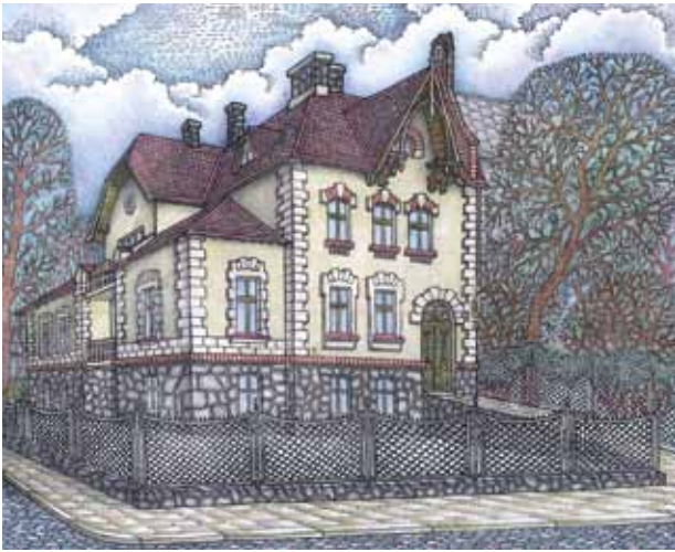
8. Colour combinations of brick and stone masonry, majolica and wooden elements in Picturesque style (4 Kolberha St.). Drawing by the author, 2016
