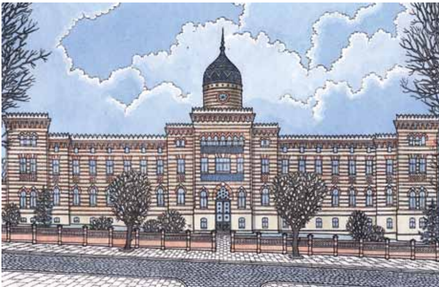
11. Opus mixtum masonry, majolica inserts and coloured roof tiles in Picturesque style (former Jewish Hospital, Rapoport St.). Drawing by the author, 2016
