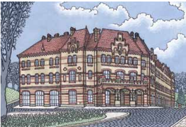
10. Opus mixtum masonry and coloured roof tiles in Picturesque style (6 Pidvalna St.). Drawing by the author, 2016
