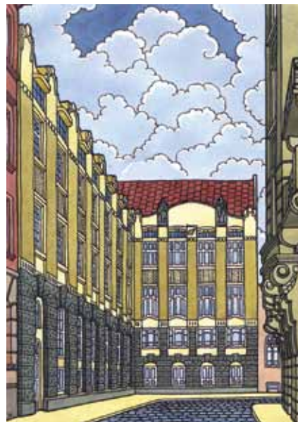
13. Faux stone socle, majolica panels, complex colour palette of a Secession façade (5 Nyzshankivskoho St.). Drawing by the author, 2016
