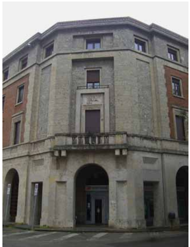
5. Edifice of the National Insurance Institute (INA) in Ferrara, photo by Blazej Ciarkowski
